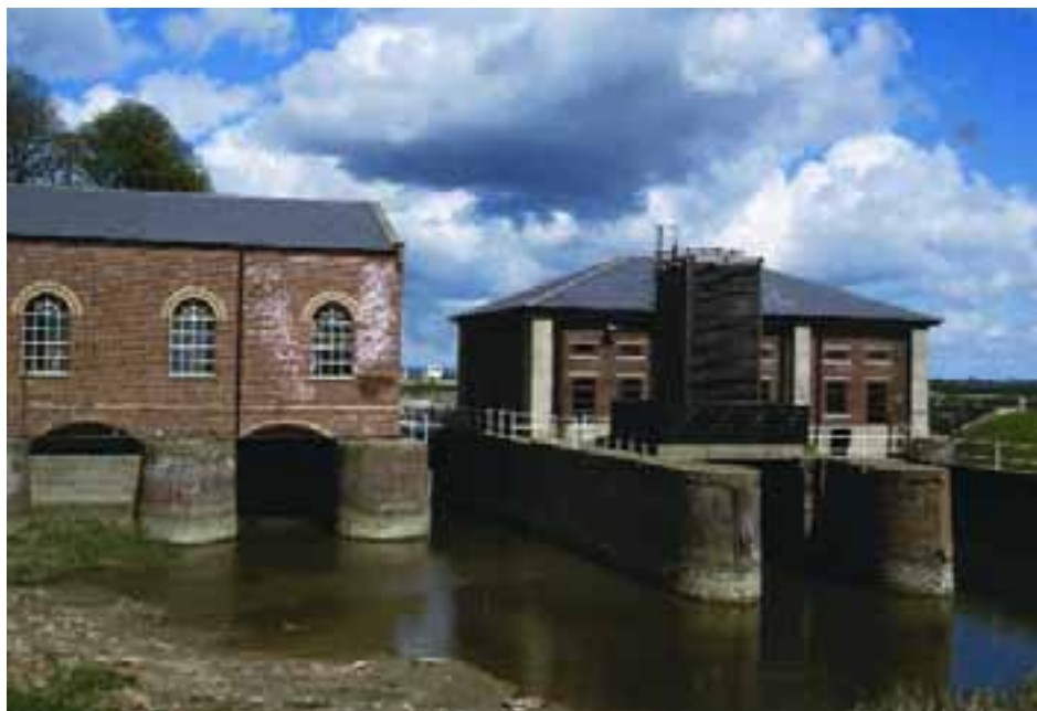
Lade Bank pumping station on Hobhole Drain
