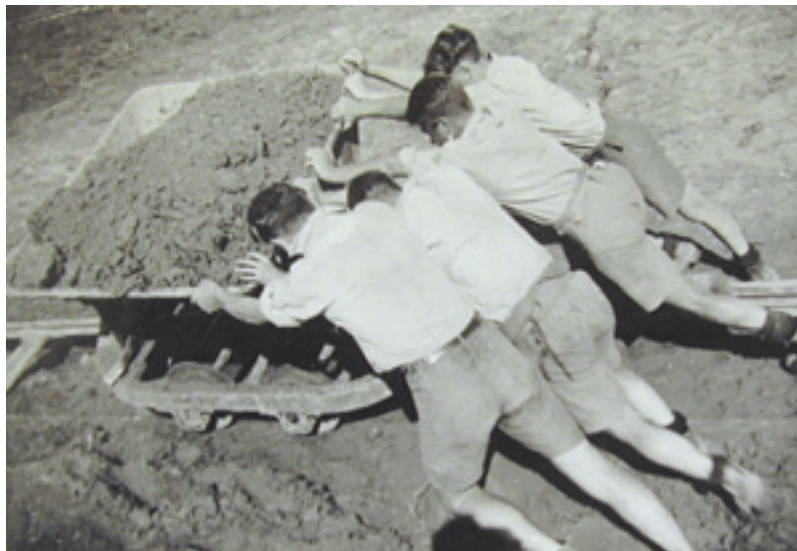
Boys undertaking the back-breaking work of creating the new sea wall
