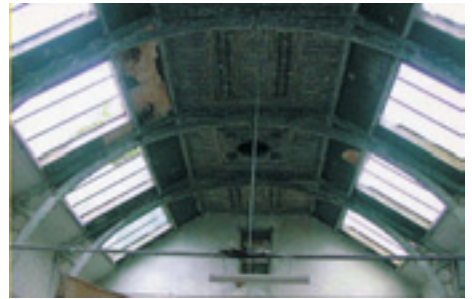
The carved, glue-laminated wooden truss supports are believed to be the earliest of their type in Britain
