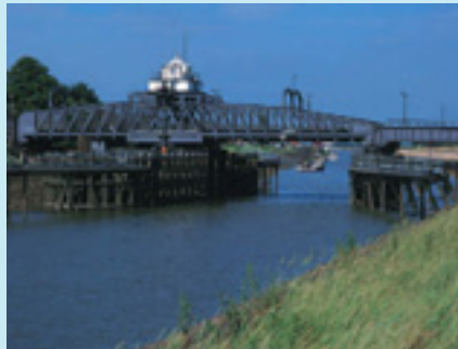
Cross Keys swing bridge at Sutton Bridge JOHN SMITH
